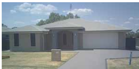
Lot 9 Layne Crescent
